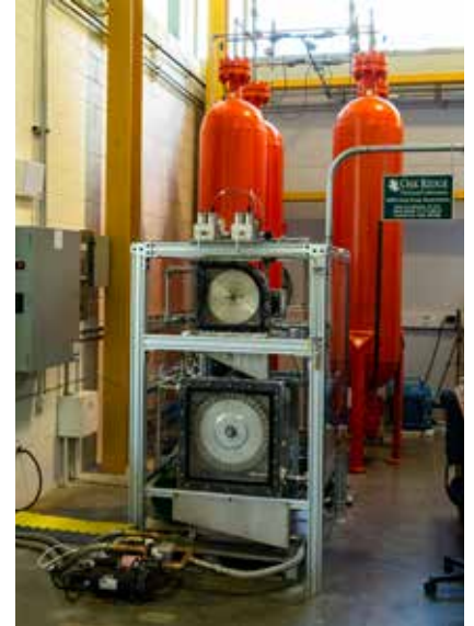
Low-cost energy storage system powered by water
