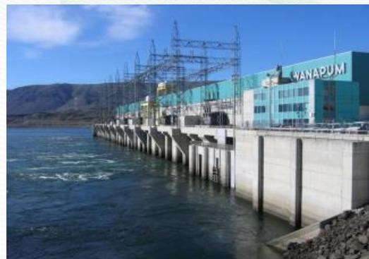
*Passage of fish through turbines, like those Wanapum Dam on the Columbia River, can cause fish injury or death via turbine blade strike, rapid pressure drops, and water turbulence.*
